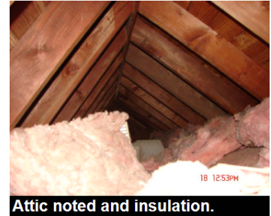
Attic noted and insulation.
